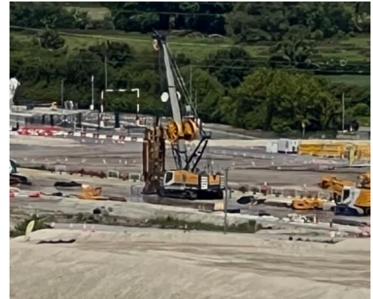
Clam Type Excavator for Permeable Wall
