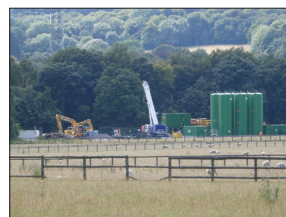
Bentonite tanks at the Small Dean Viaduct piling site
