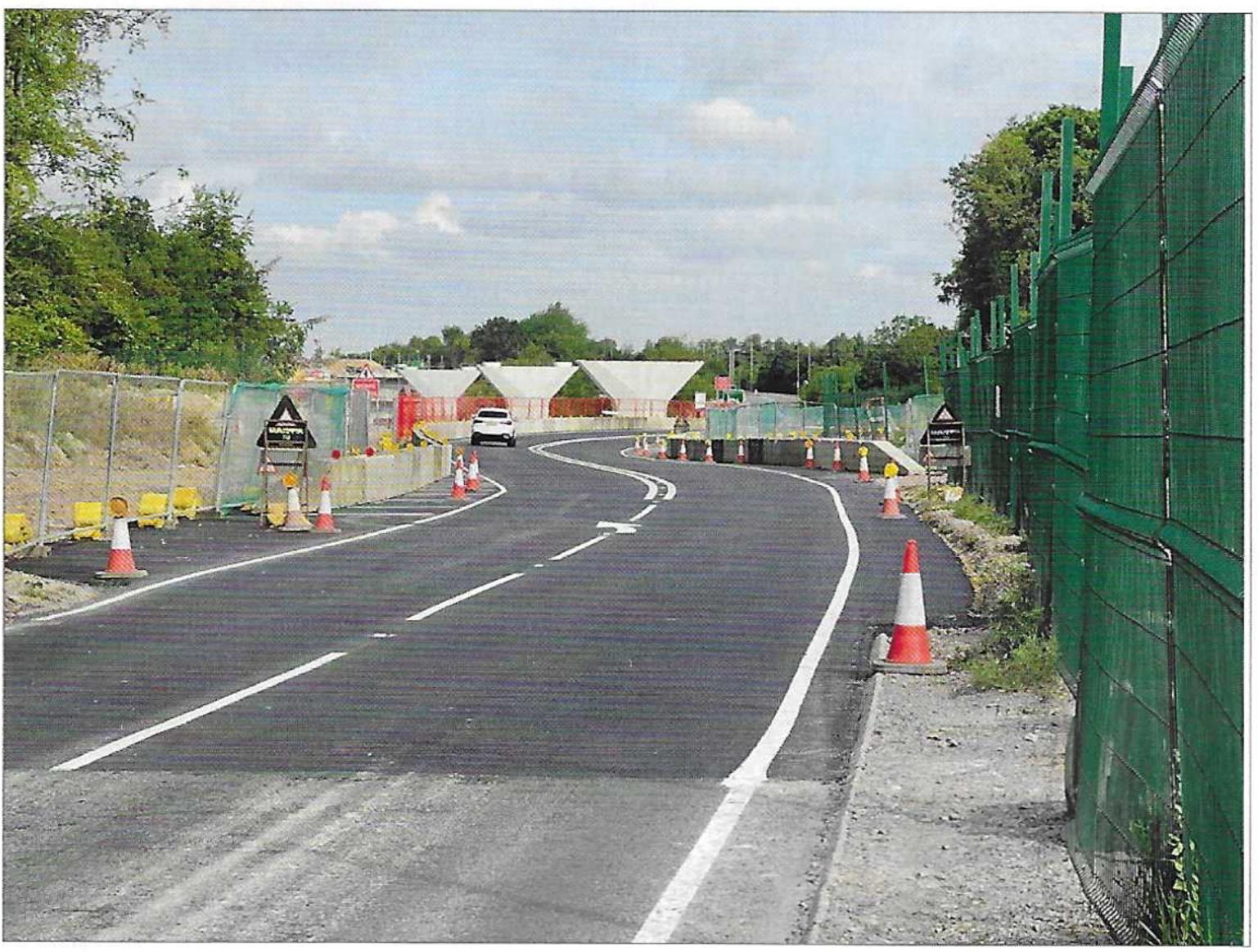
The road currently bends sharply around the site, but this will be smoothed out following the completion of the viaduct deck next year. The 40mph speed limit will be retained, however. The three inverted triangular structures in the middle of the photograph above are the completed piers which will eventually support the viaduct.
