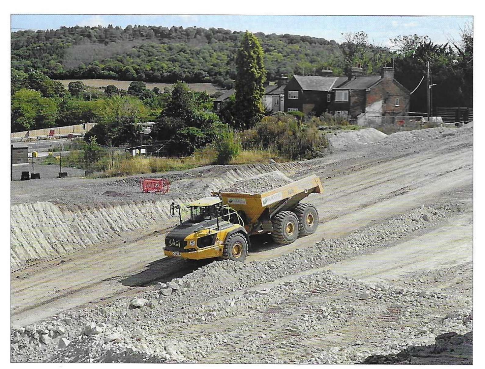
will probably continue to the end of next year. The massive Volvo dump trucks can carry up to 60 tons of spoil and are surprisingly quiet. However, the tracks of the bulldozers used to level out the stockpile are certainly audible in Wendover when the wind is from the west. Monitoring of the noise, vibration, and air quality is undertaken at Ellesborough Road and so far the results are within the limits agreed with the council.
