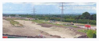
North Cutting up to Nash Lee Road will start next year, following the installation of the tanking wall to stop aquifer water pouring into the works.
