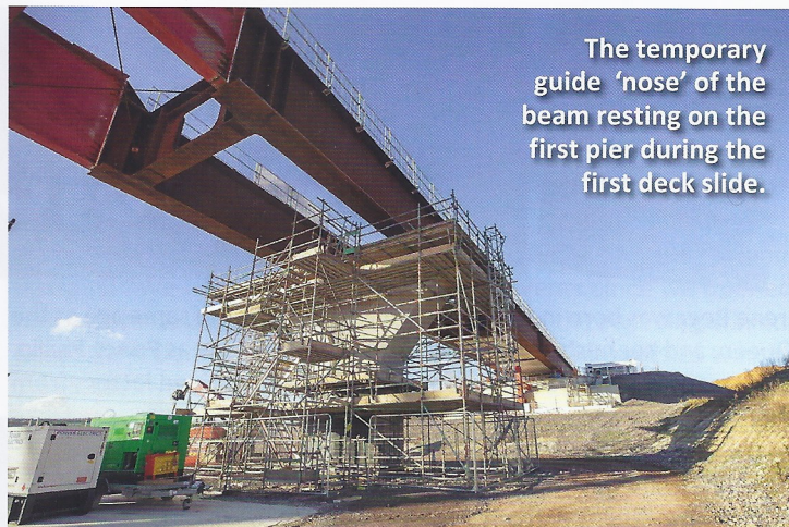
Specialist engineers from Eiffage Metal carefully guide the sliding deck into position.
