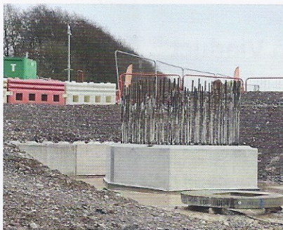
A pier foundation such as this will soon be constructed adjacent to the newly aligned A413 London Road
