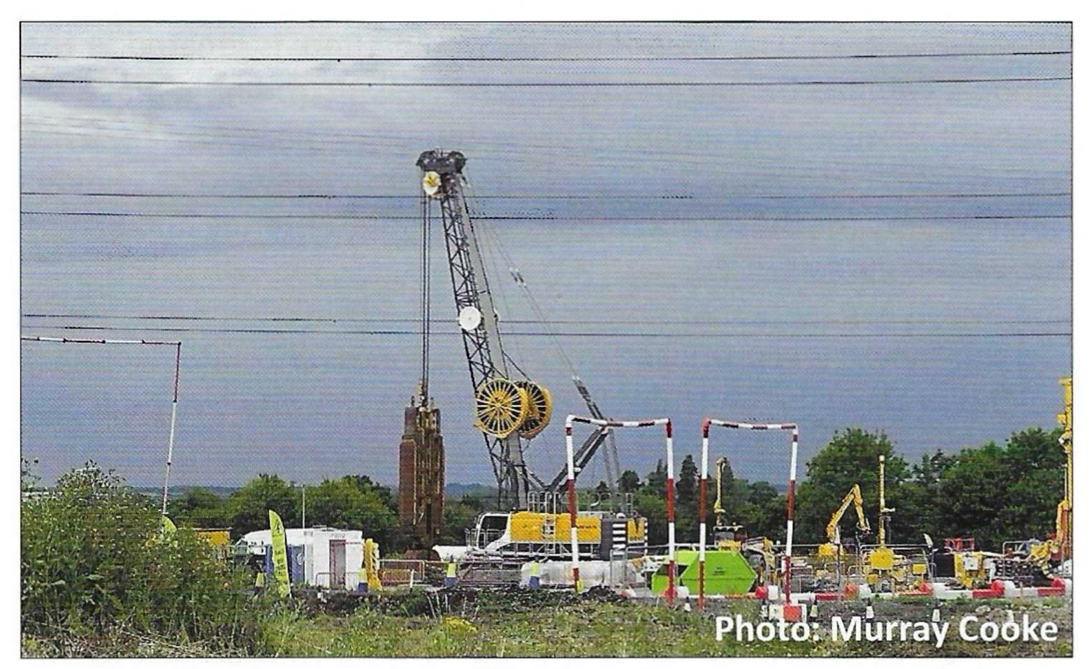
The 30m deep trenches will be dug using computer-controlled excavators such as this, shown near the Nash Lee end of the site
