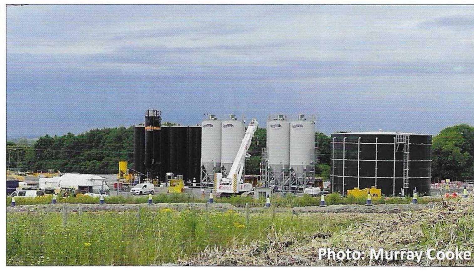
Pouring concrete for the underground wall is time-critical. The mix will be prepared on-site using the new concrete slurry batching plant
