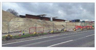
Meanwhile the steel deck sections are being welded together before being launched over the piers next year.
